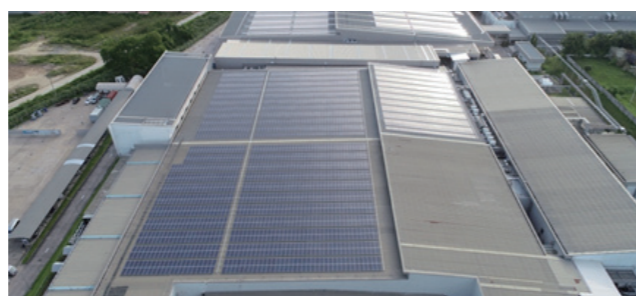
Mega solar panels installed at TRT (Thailand)
