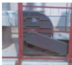
▲活性炭吸着装置 Activated-charcoal adsorption unit
